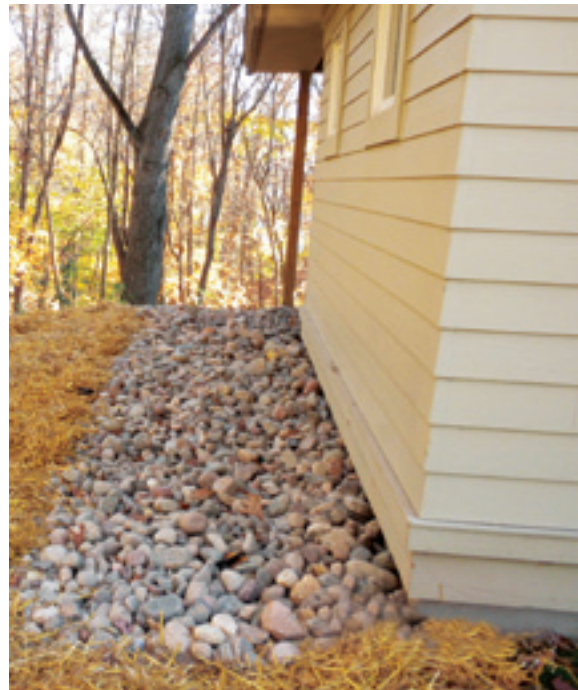
Nancy Deschane and Dean Sather's gutterless garage was causing erosion, so they installed a rock trench to catch and infiltrate water.
