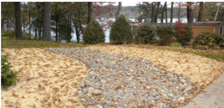
Areas filled with rock are another option for creating water storage to alleviate erosion by filtering water runoff from roads and driveways.
