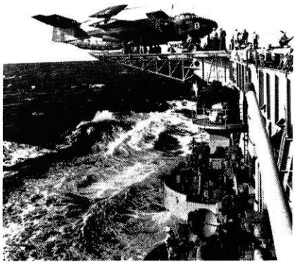
Deck-edge elevator on the carrier Midway.
