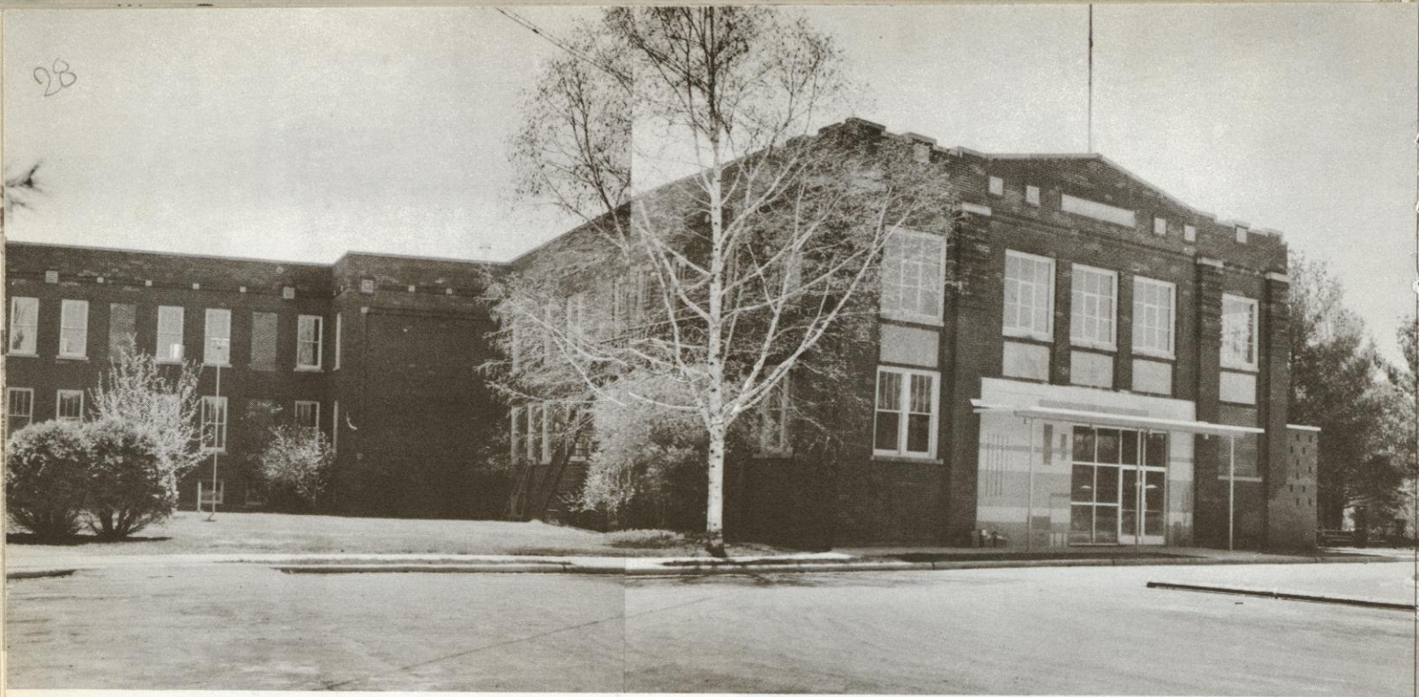
REMODELED QUARTERS FOR SANATORIUM -- This structure, formerly known as the Willard Preventorium, is now Mt. View Sanatorium. The building, formerly used for children who contracted tuberculosis, has been completely remodeled by Marathon County and is now serving its capacity of about 33 patients. Miracle drugs have helped cut down the number of TB patients. At one time the main sanatorium (shown on opposite page) and the preventorium had a total of 90 patients.
