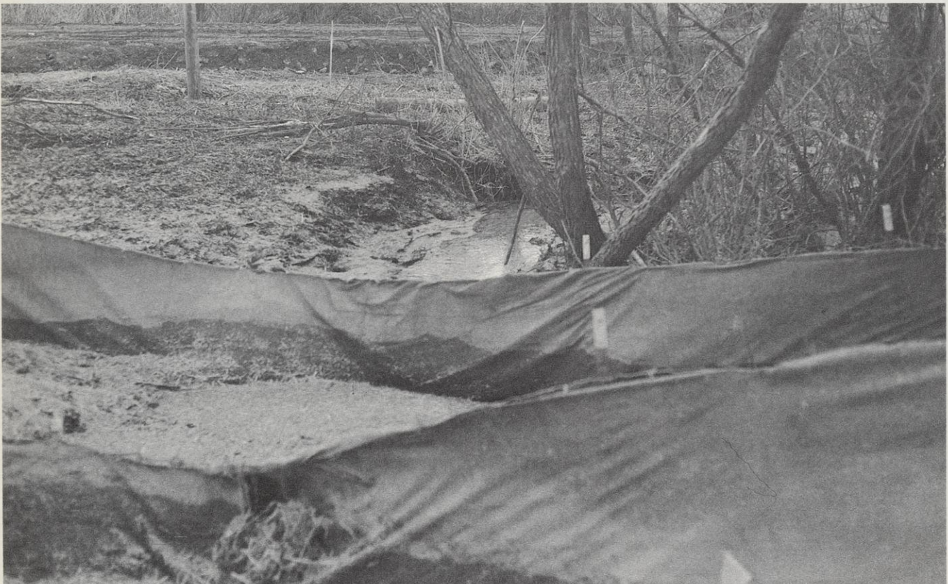
Filter fabric controls construction site erosion by trapping sediment. Strawbales, sodstrips, seeding and mulching also work. Photo by Jim Baumann
