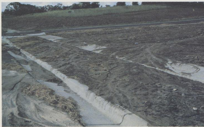
The okay and the bad at two construction sites. Straw bales at one hold back sediment and protect receiving waters. The other messes up the street and fills the storm sewer. Actually, the bare soil on both should have been protected. Photos by Susan Bergquist
