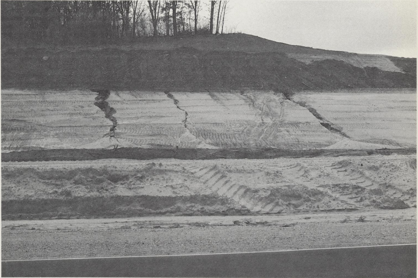
Typical highway construction scene. Raw roadbeds and banks are often left exposed for months. Rapid soil stabilization and revegetation are needed, coupled with water detention strategies, to protect receiving waters and avoid costly cleanup. Photo by Susan Bergquist
