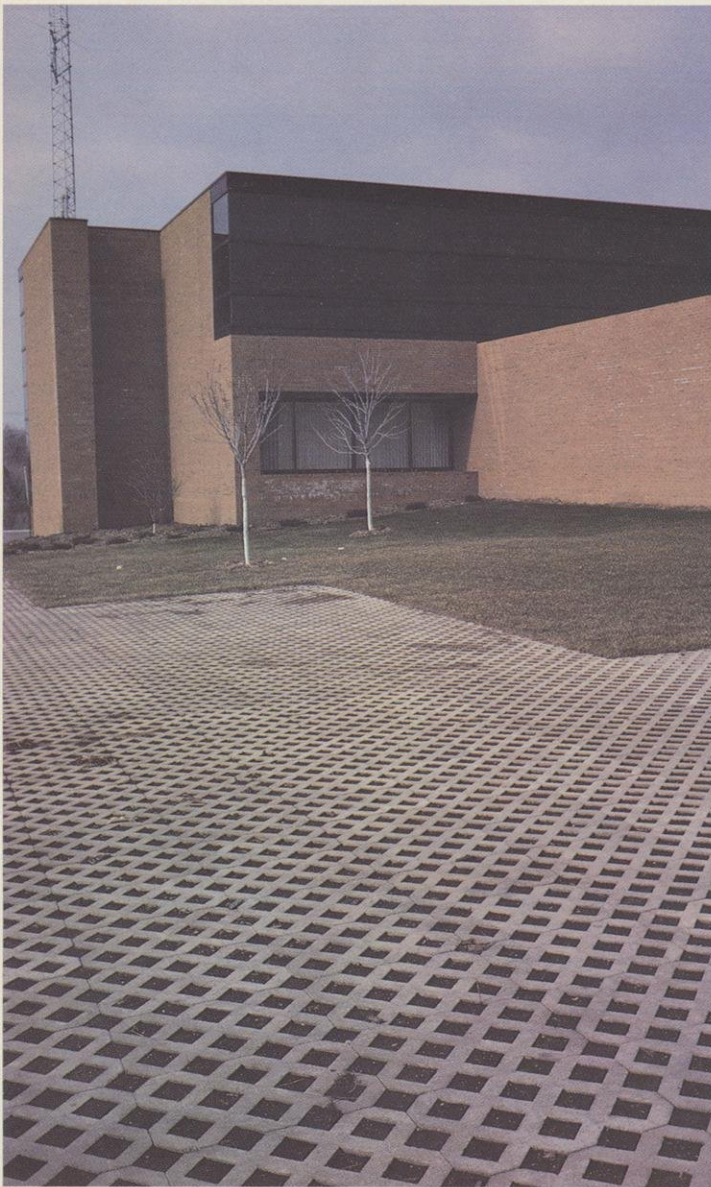
Porous pavement provides a hard surface yet allows infiltration of water. The openings can be planted with grass or filled with loose material. Photo by Robert Pitt
