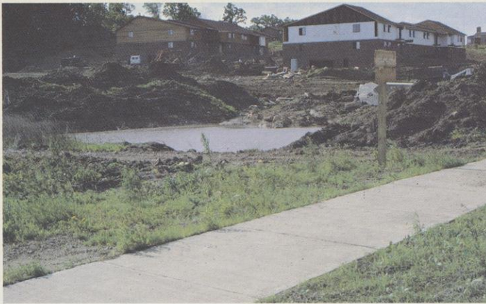
Detention basins can trap runoff and sediment during construction, then later be attractively incorporated into landscape design and continue to serve the same function. This is a condominium project in Madison. Photos by Susan Bergquist
