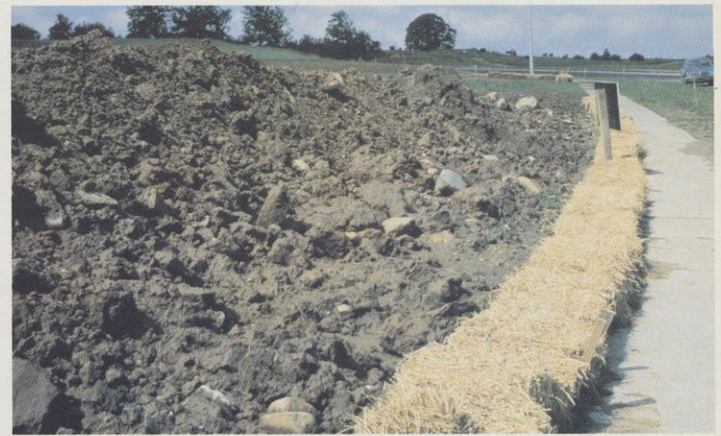
The okay and the bad at two construction sites. Straw bales at one hold back sediment and protect receiving waters. The other messes up the street and fills the storm sewer. Actually, the bare soil on both should have been protected. Photos by Susan Bergquist
