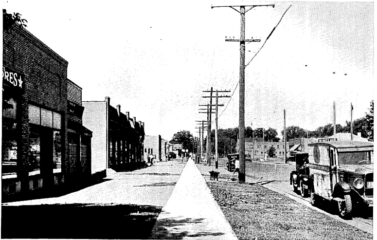
City planning. Through the use of set-back building lines, major streets can be progressively and economically widened. Note the new buildings on the left side of the street set back on the proposed new street line.
