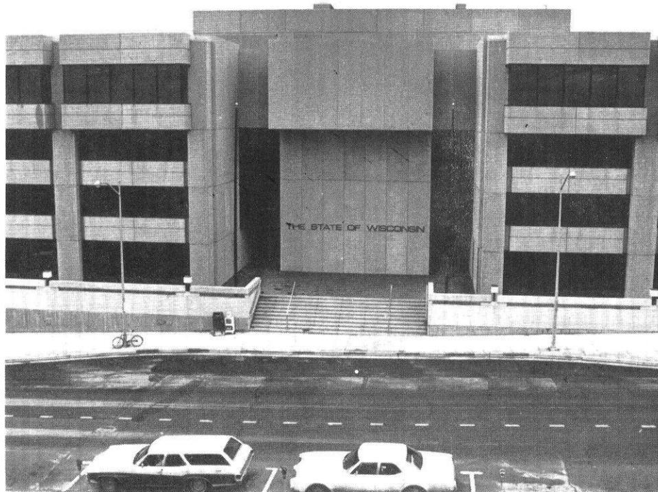
Lighting problems originally plagued a new Wisconsin state office building. Due to a computer breakdown, lights burned 24 hours a day.
