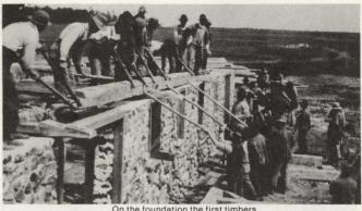
them with little braces, girts, and storm braces were razed. When they were all razed, the frame work of the structure was finished. The most dangerous job was about to take place. The perline plates with posts and braces were joined and put on top of this structure. When that was all joined and finished the
