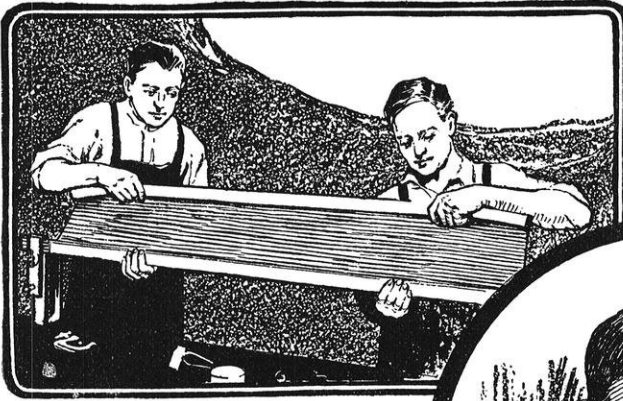
Winding high voltage insulation, 1894— 2,200 Volts
