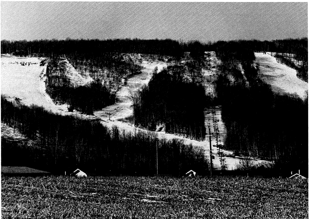
Fig. 6. Rib Mountain Ski Area, from the north.
