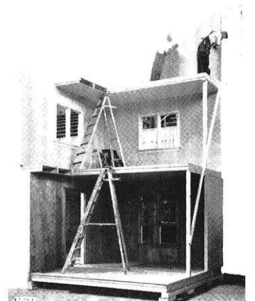
FIG. 6—Erecting attic panels.
