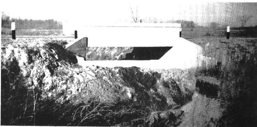
Treatment of culvert to stop gully from advancing.
