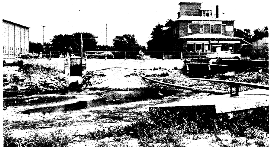
FIGURE 4 The Marion dam showing the emergency wasteway and flume (looking east).
