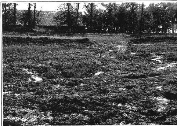
This picture shows a terrace outlet before construction of sod channel.
