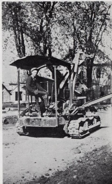
Barney Diederich operating the Back filler while laying the water works and sewer system in 1927.
