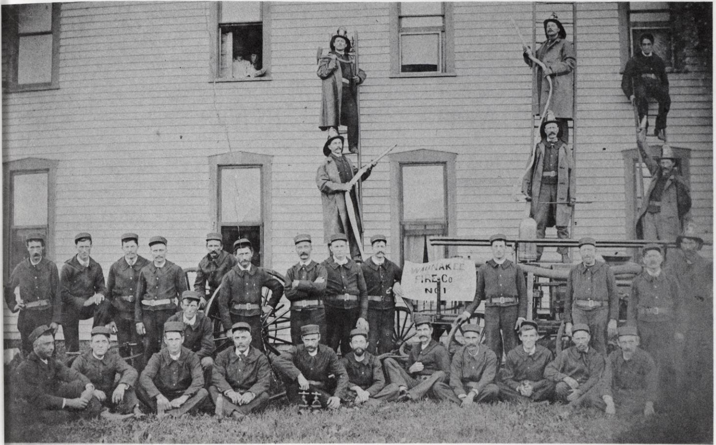
Earliest Picture taken of Waunakee Fire Co. Taken along side of the American House.
