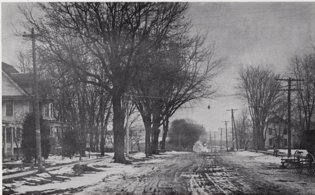
Typical view of what Main Street looked like before the paving was done. This is looking East from the McWatty house.
