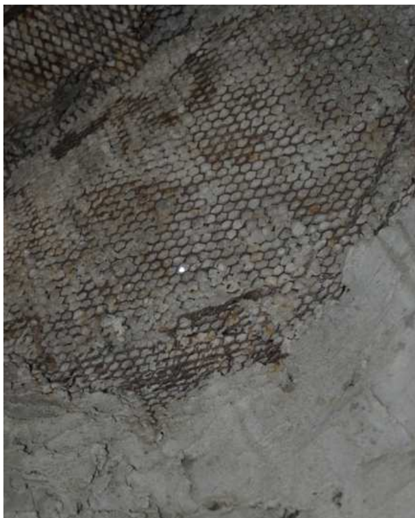
Figure 4.5: James Tellen, detail of cement reinforcement, Woodland Sculpture Garden , Black River WI, 1942-1957
