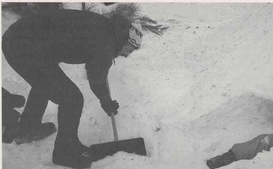
Diggers carefully hollow out a thick wall in the hardened shelter, scooping snow out the entryway where others shovel it away.
