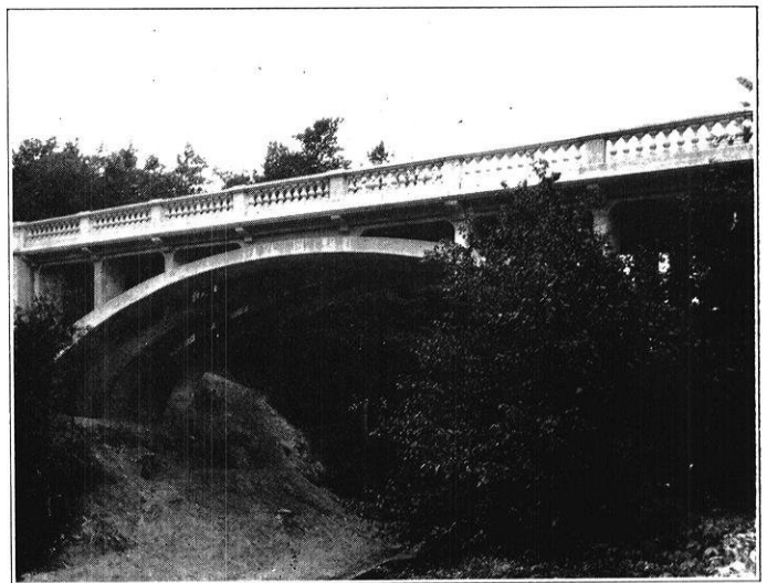
The construction features such as the triple arch, open spandrels, and decorative railing, are visible in this view taken from below the bridge near Eau Claire, Wisconsin. It was built two years ago, under the direction of the Wisconsin Highway Commission.
