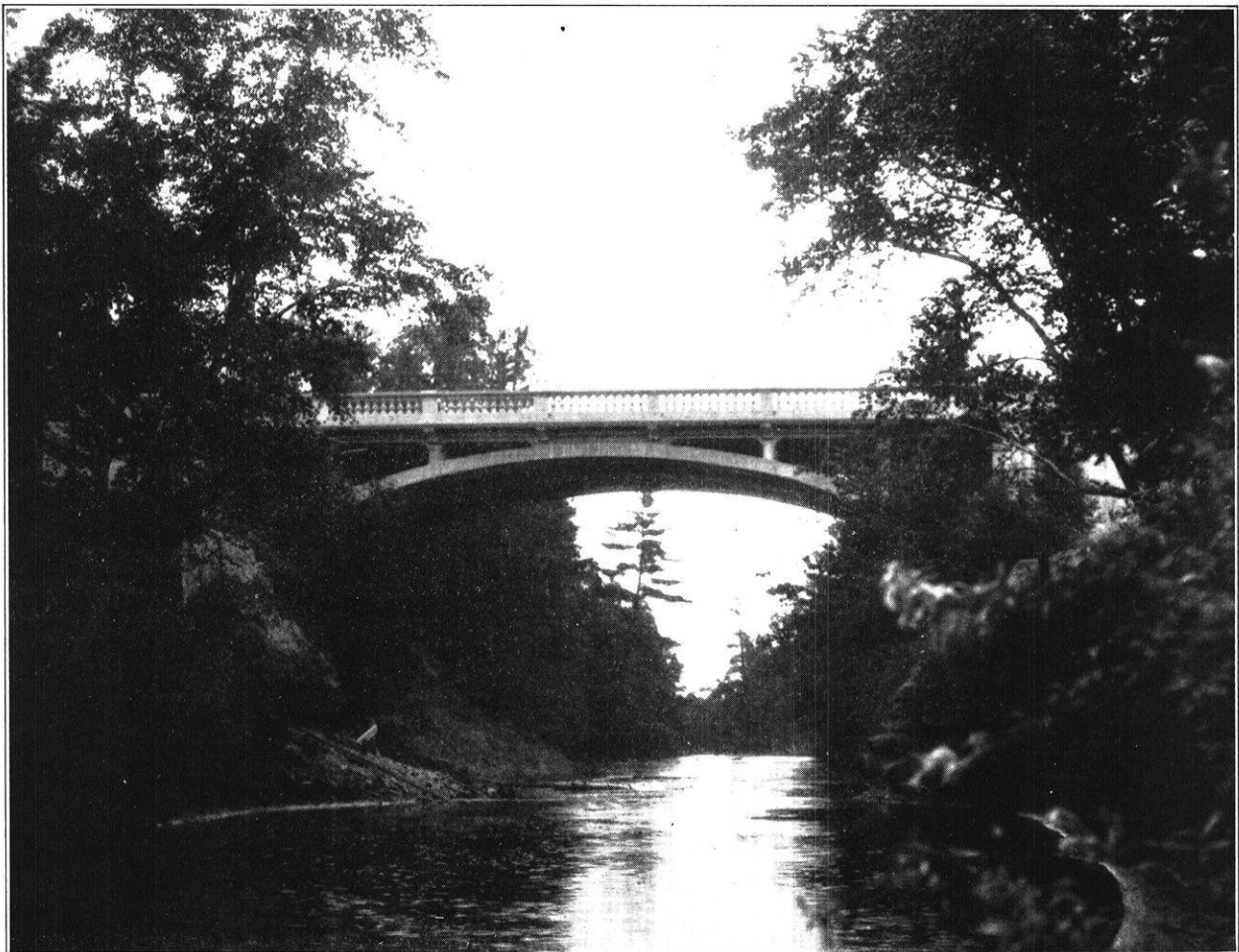
OTTER CREEK HIGHWAY BRIDGE
