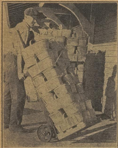
Trucking 6-qt. baskets with a Lizzie truck. Note how it saves labor. It has been proposed that the Dominion Government shall standardize this basket.
