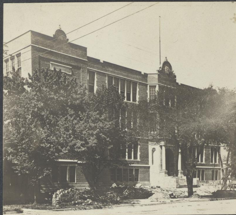
21-M.H.S. in Course of Construction.
