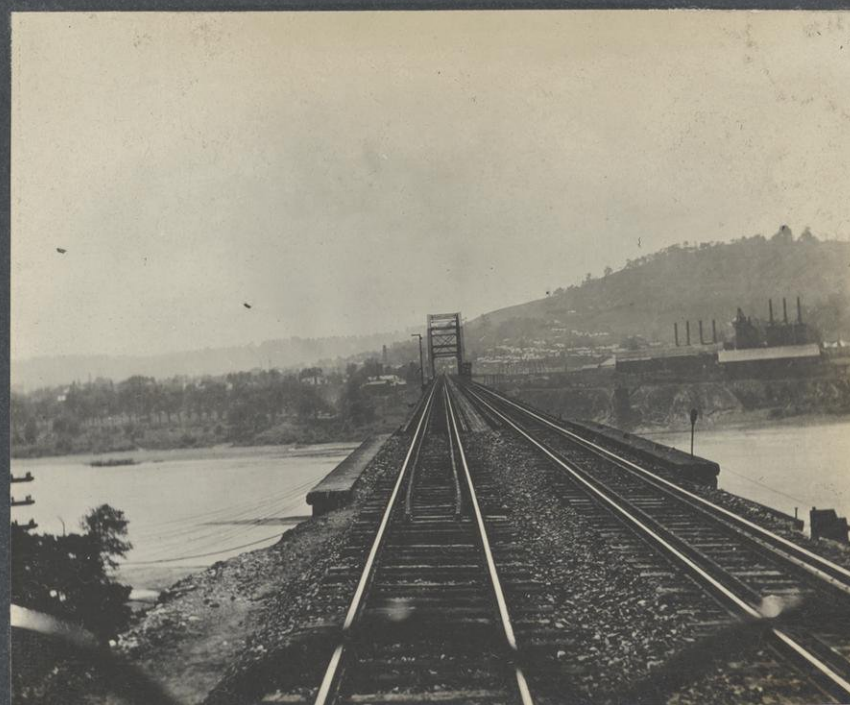
95 - Pa. Ry. Bridge over Ohio R.
