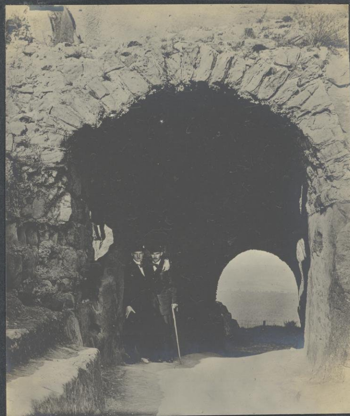
136-A Tunnel, Regenstein-West & Chaney.
