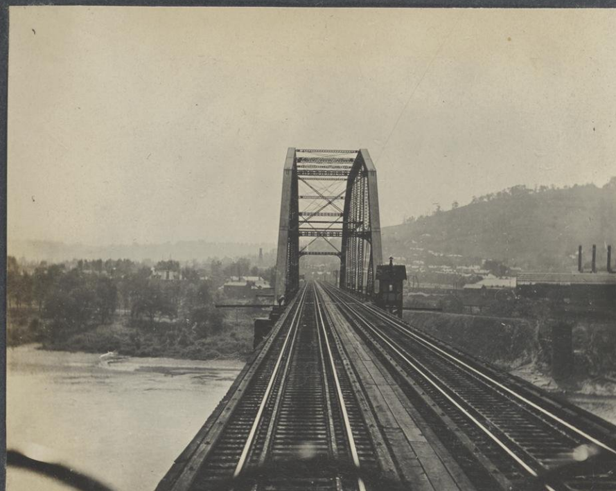
94 - Drawbridge of Pa. Ry. over Ohio R.
