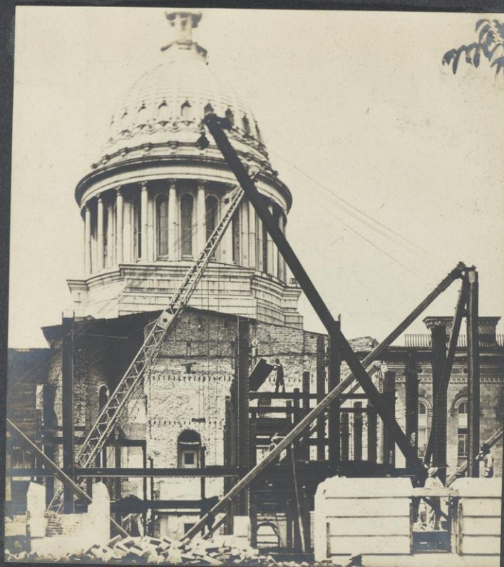
12 - Big Derrick Placing Load.
