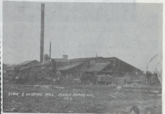
STAVE & HEADING MILL
