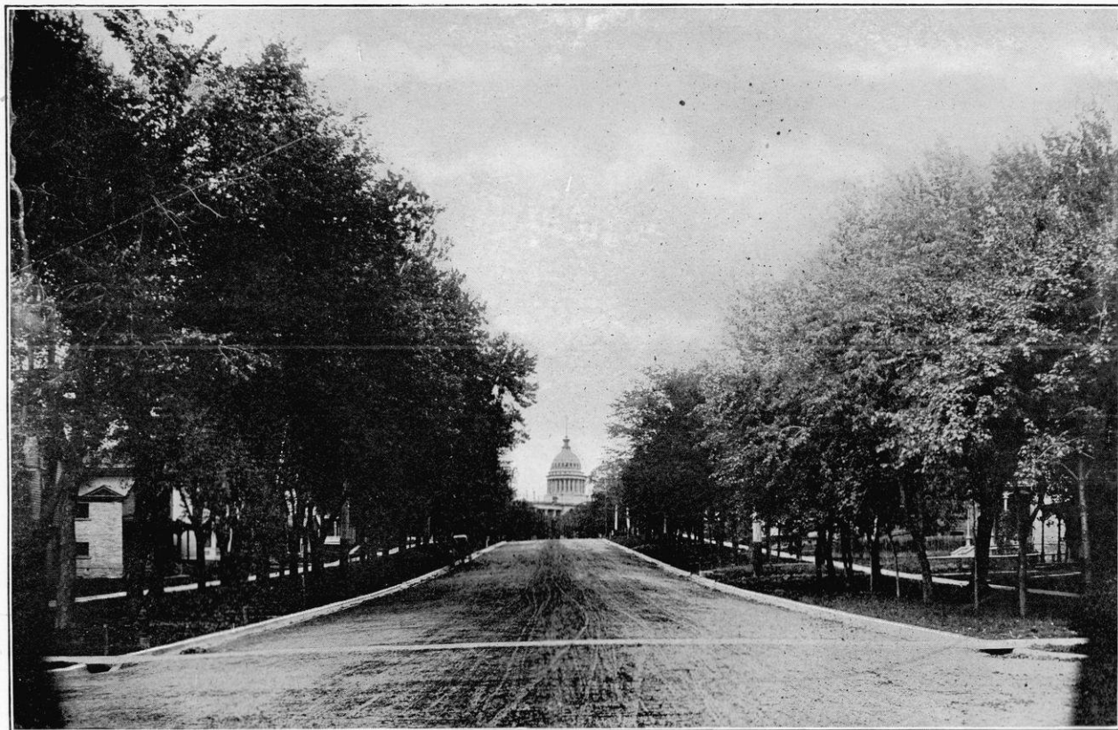
Limestone Macadam Pavement. New. West Washington Avenue, Looking Northeast from Broom Street, Madison, Wis.
