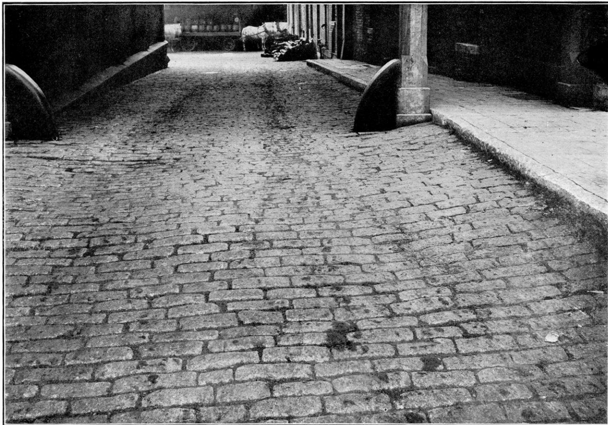
Granite Block Pavement. Entrance to Pabst brewery. Heavy traffic. Compare with pavement illustrated on opposite page.
