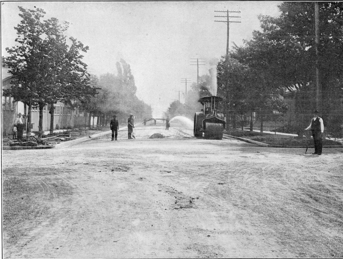
Bonding the Macadam Pavement, Michigan Avenue, Sheboygan, Wis.
