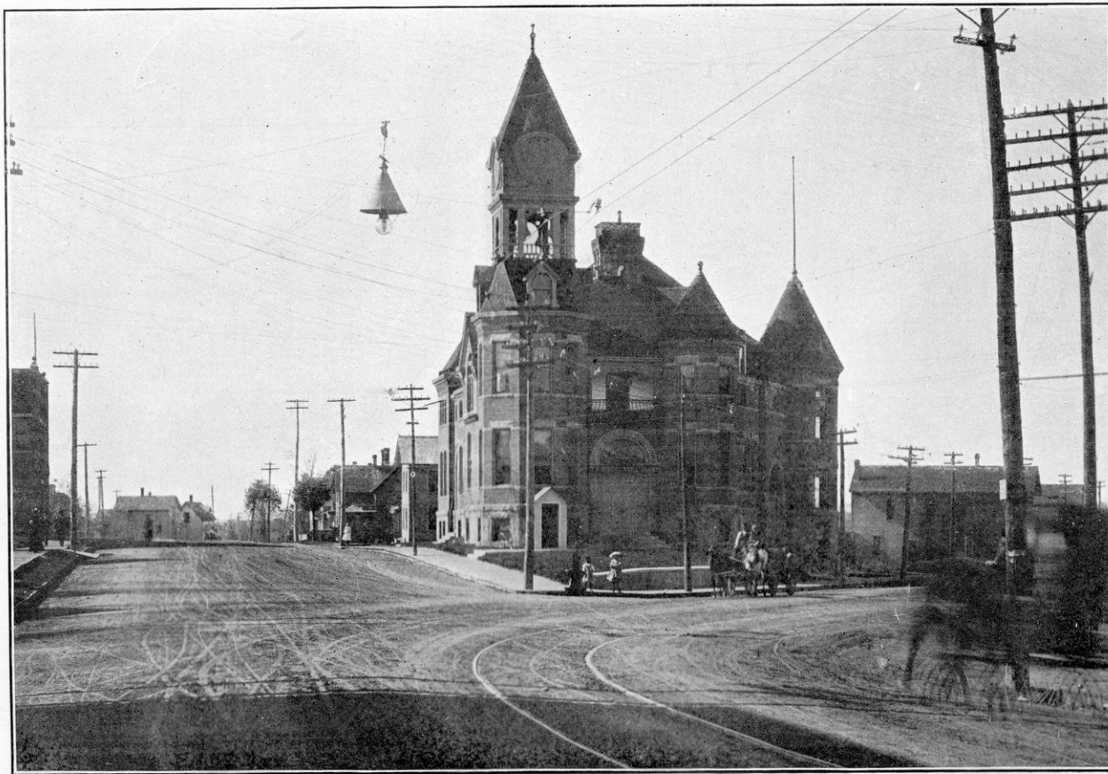
Macadam Pavement, Merrill, Wis.
