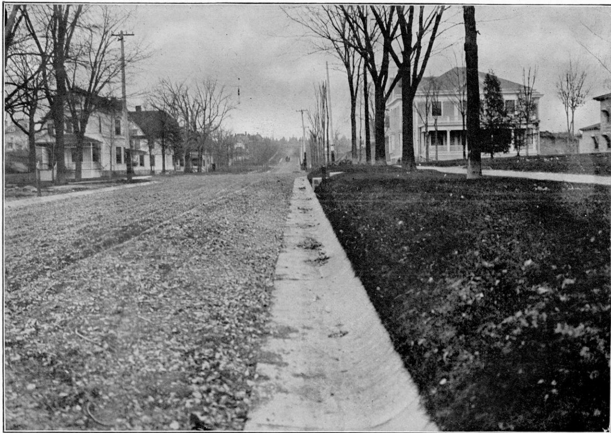
Cement Gutter without Curb, Ash Street, Baraboo, Wis.
