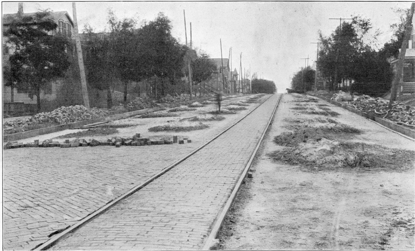
Brick Pavement Partly Constructed. North Main Street, Racine, Wis.
