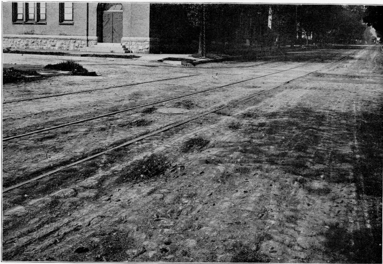
Cedar Block Pavement. Wells Street, between Sixteenth and Eighteenth Streets, Milwaukee, Wis.
