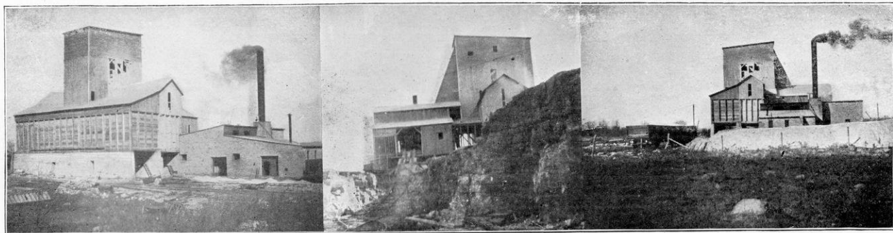
Crushing Plants, Lannon, Wis.
