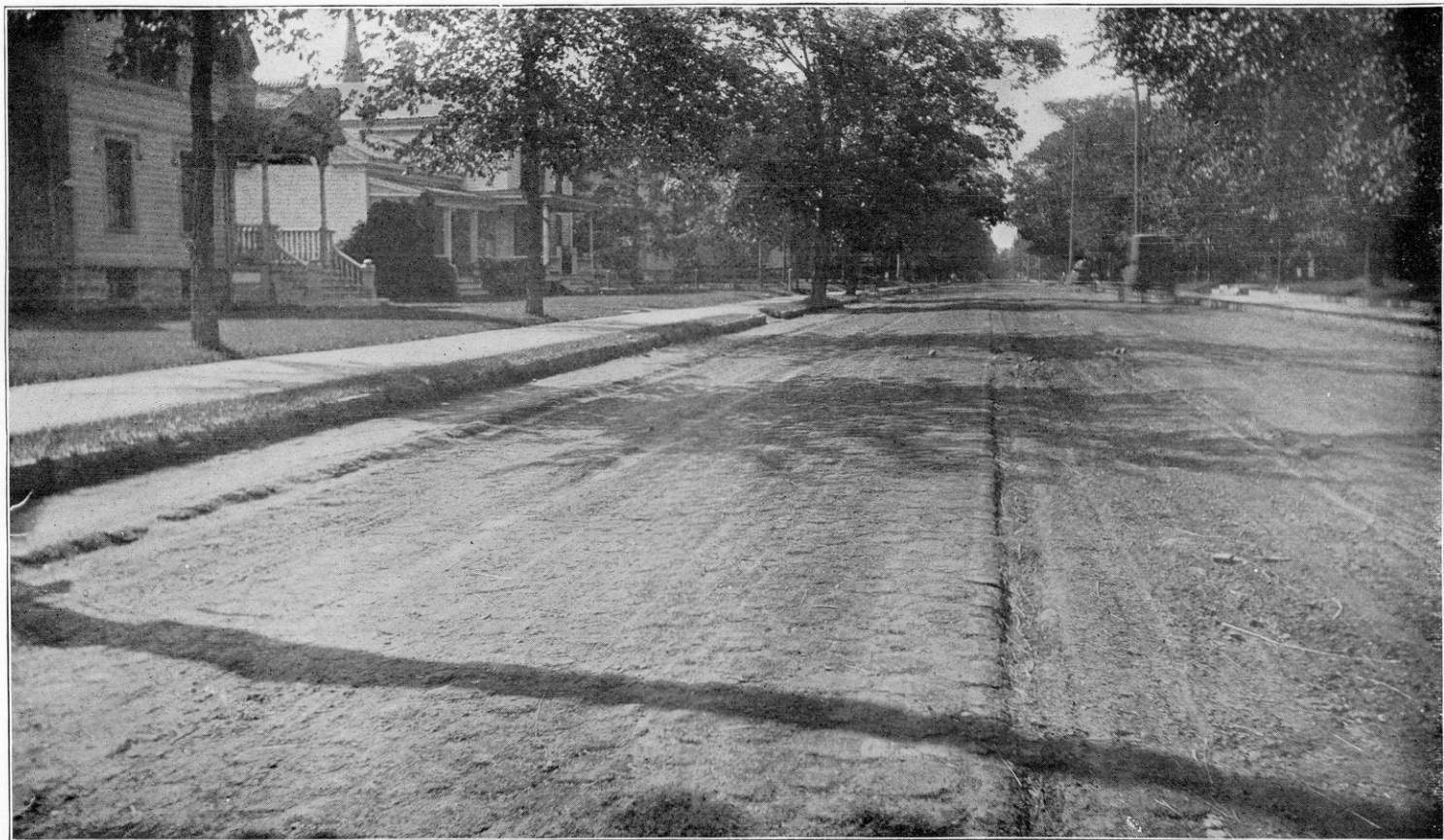
Cedar Block Pavement, Showing Removal of Street Car Tracks. Algoma Street, Oshkosh, Wis.
