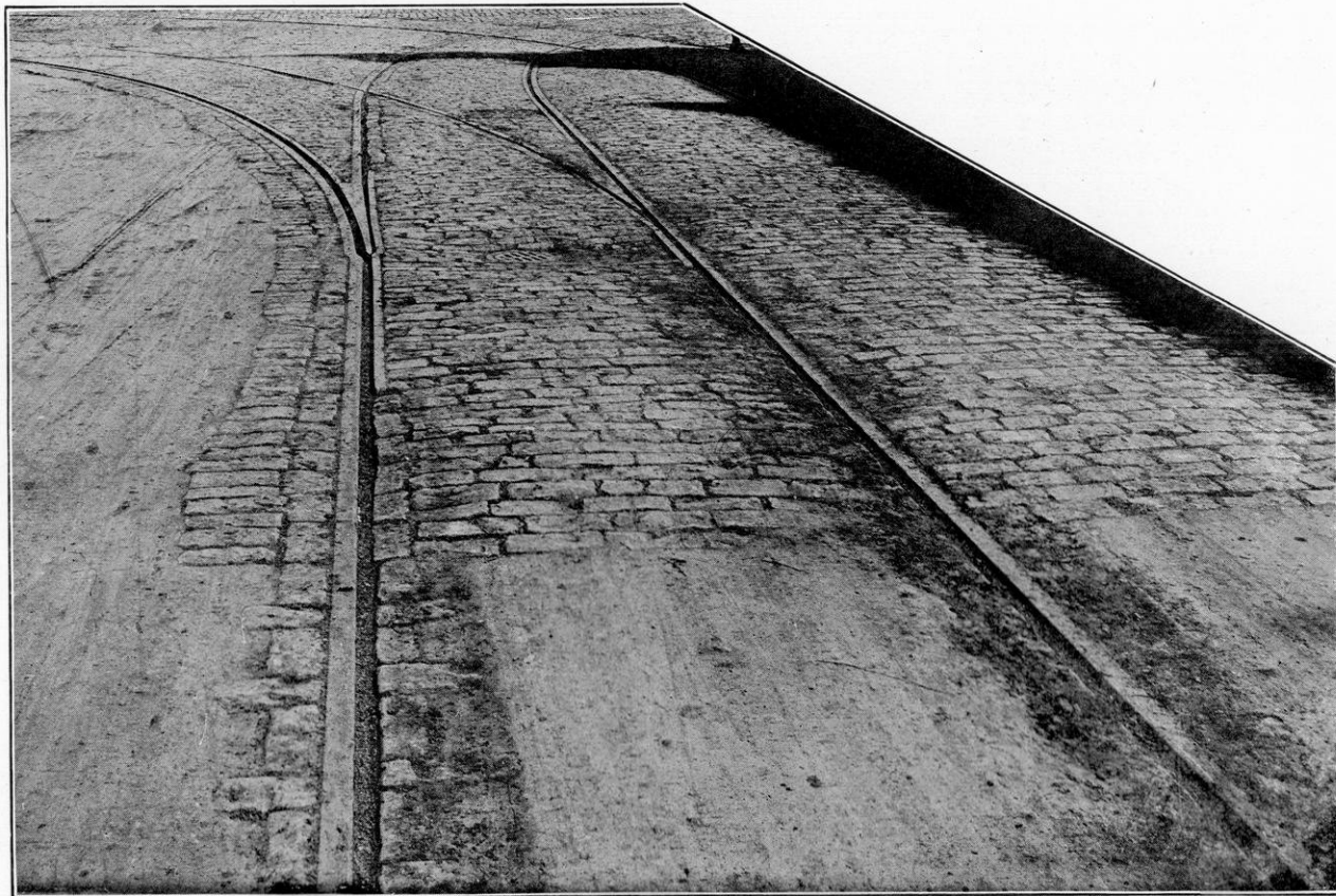
Asphalt Pavement. Intersection of East Water and Oneida Streets, Milwaukee, Wis. Showing use of granite blocks between the street car tracks.
