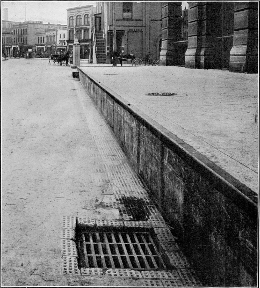
Brick Gutter, Cement Curb and Granolithic Sidewalk. Second Street, Milwaukee, Wis. Corner of curb protected with steel plates.
