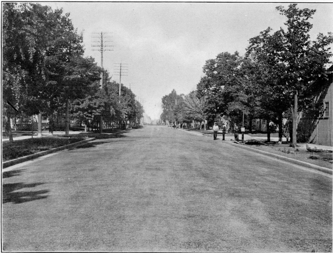
Granite Top Macadam Pavement. Michigan Avenue, Sheboygan, Wis. Built in 1901.
