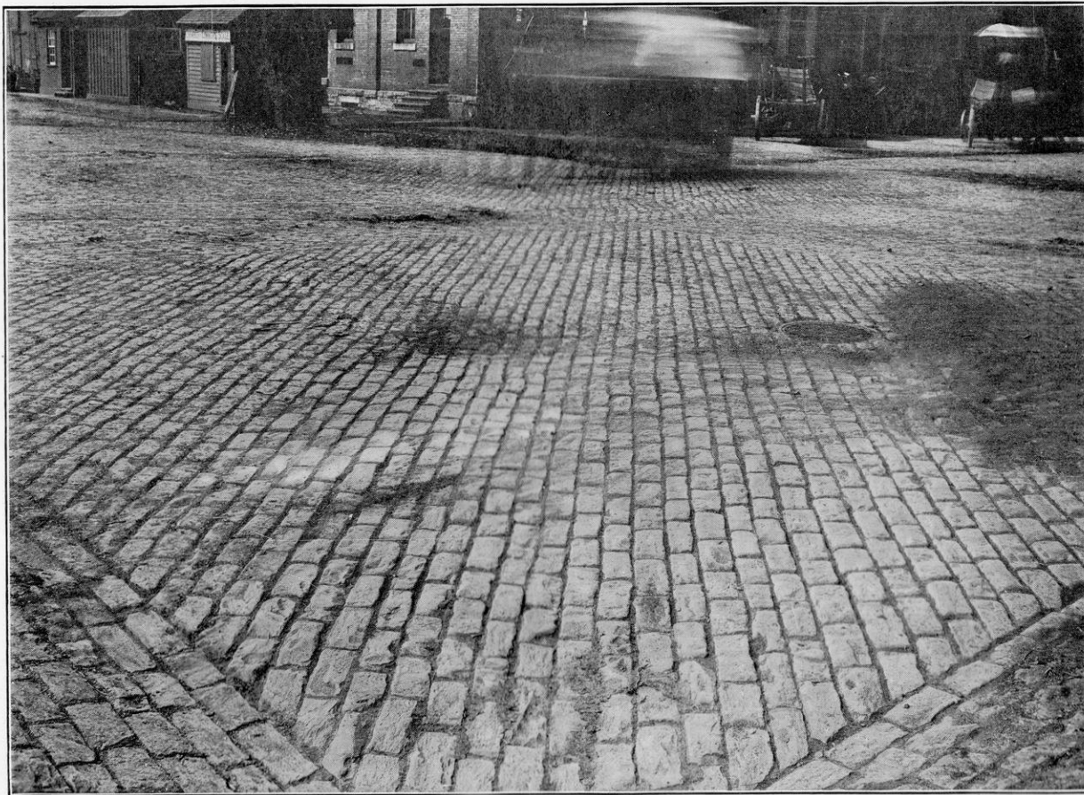
Granite Block Pavement. Intersection of Second and Fowler Streets, Milwaukee, Wis.
