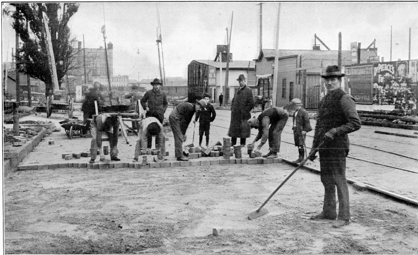
Brick Pavement in Process of Construction. North Main Street, Racine, Wis.
