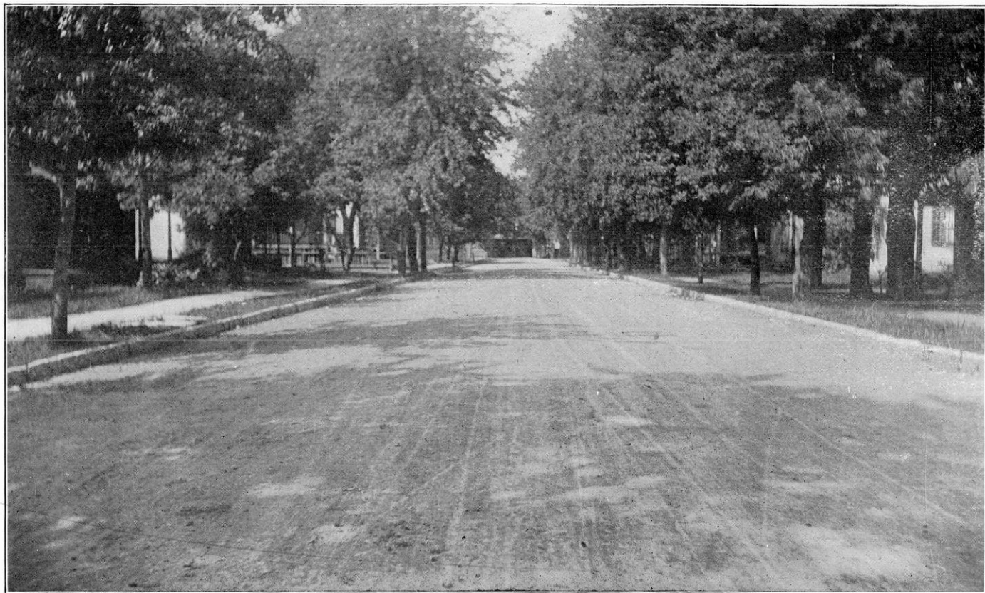
New Limestone Macadam Pavement. Pleasant Avenue, between Merrit and Hudson Streets. Oshkosh, Wis.
