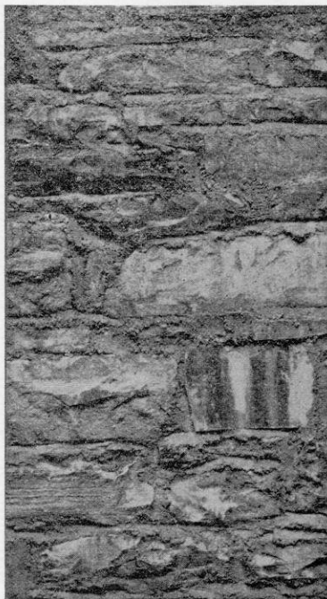
Stone Work of Exterior
