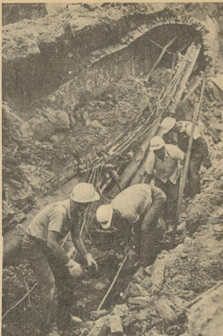
ANYONE SEEN MY CONTACTS?—Workmen at the Historical Library construction site uncover a telephone cable that was severed about 6 p.m. Wednesday. Service to lower campus buildings, including the Union, was cut. Telephone company crews worked through the night to replace 15 feet of cable that was damaged.
