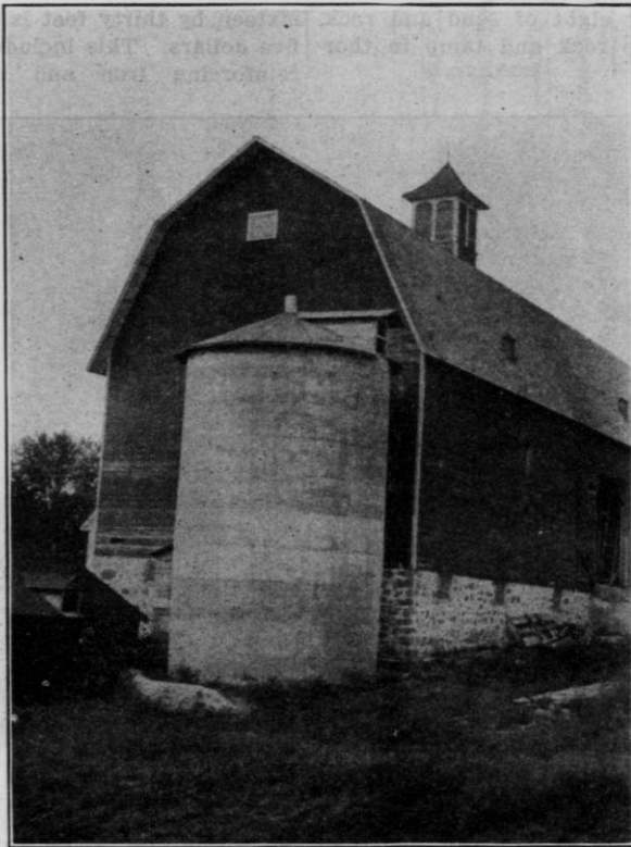
John Imrie's concrete silo completed.
