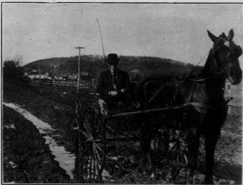
North Freedom road before improvement after a rain.
