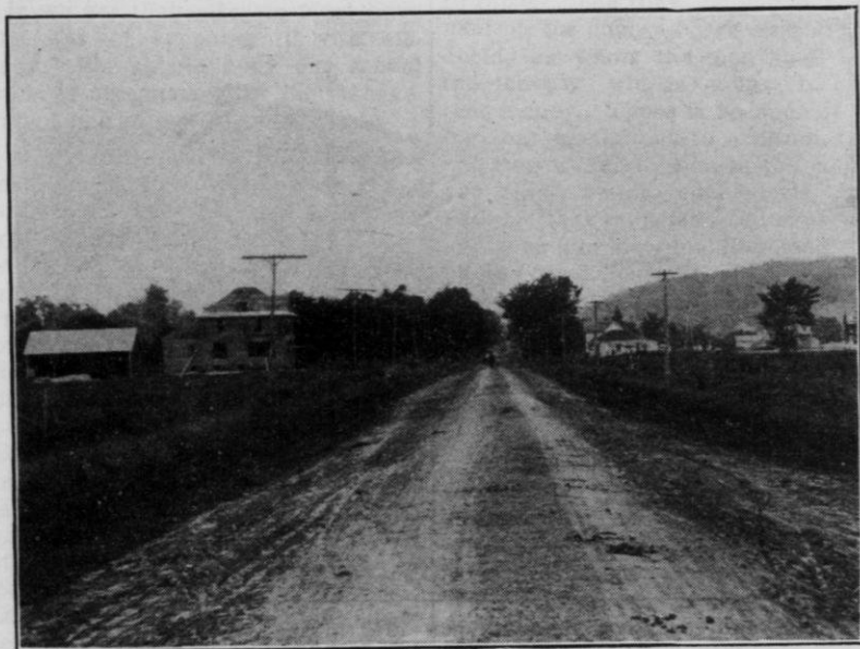
North Freedom road after improvement under county aid. Cost of this road about $2200 per mile.
