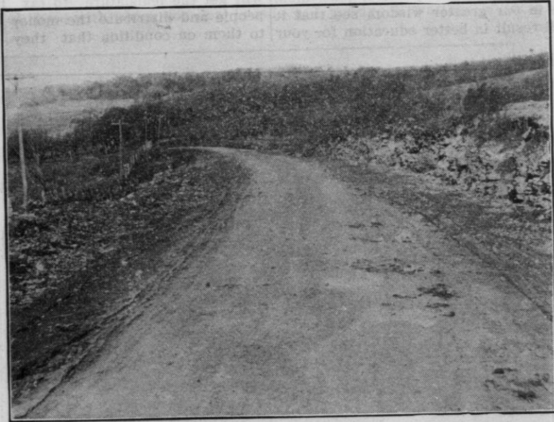
West Sauk road, Town of Baraboo, Sauk Co., showing effect of relocation. Note the old road in upper right hand corner. Steepest grade on old road 12%, on new 7%. Surveyed and planned by the Highway Division, as have all macadam roads built in Sauk Co. in 1909 and 1910. Mr. J. T. Donaghey, the County Highway Commissioner, considers rightly that surveys are in most cases necessary to obtain the best results in county road construction.
