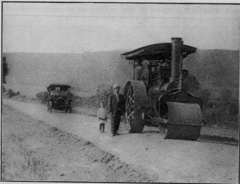
County and macadam road built in 1910 in the Town of Sumpter, Sauk Co.
