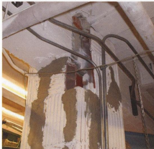
Image, bottom: Typical damaged or removed clay tile fireproofing around the pan-joist longitudinal bar.
