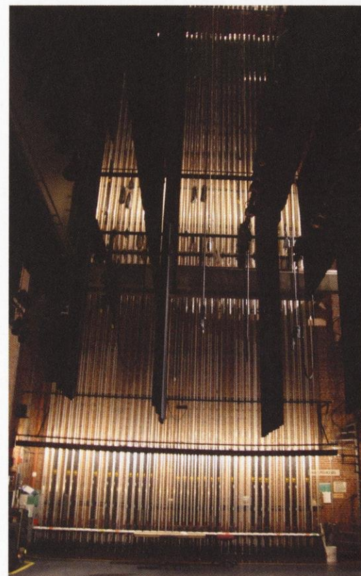
Image: View of the stage looking east with the manual counterweight rigging system visible in the background.
