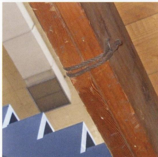
Image: Questionable cable support hanger bottom attachment in backstage area.
