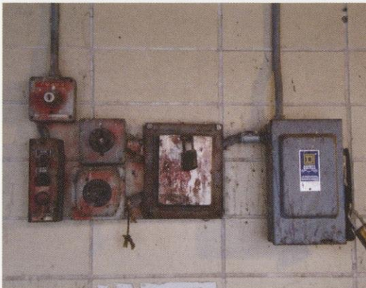
Image, top: Vintage electrical panel board and disconnects at the Union Theater stage area.
