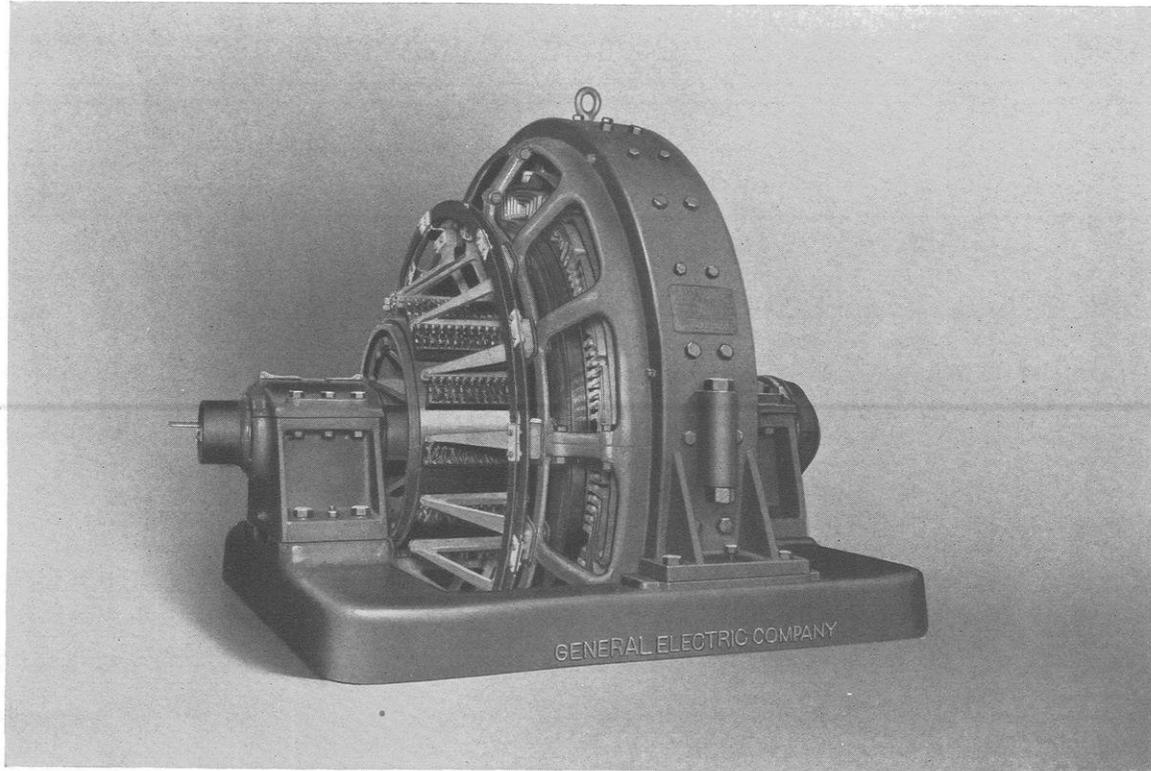
Direct-current motor, 14 pole, 2,600 h.p. Courtesy of the General Electric Company
