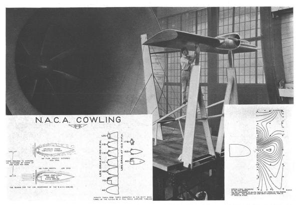
COWLED ENGINE NACELLE LOCATION TESTS IN THE N.A.C.A. 20-FOOT WIND TUNNEL Effect of cowling a radial air-cooled engine and determination of the most efficient arrangement of a propeller, cowled radial engine, nacelle, and wing in combination
