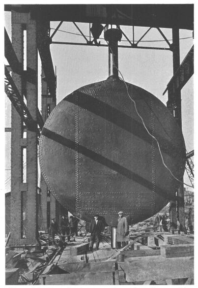
Niagara Falls. Butterfly valve to control water flow. Courtesy of the Niagara Falls Power Company
