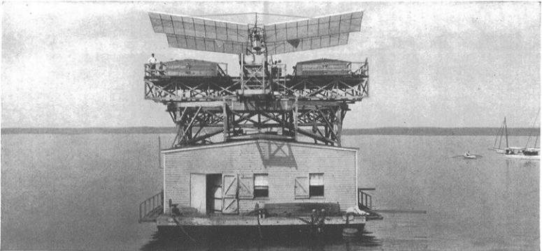
Upper: Manly 52-h.p. radial gasoline engine, built for Langley's full scale airplane. Weight 120 pounds. Lower: Langley's full-scale airplane poised for flight
