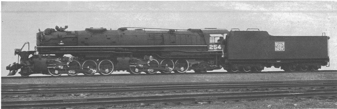
Upper: Heavy-duty passenger or freight engine. Total weight 408,000 pounds. Boiler pressure 250 pounds. Heating surface 5,422 square feet. Tractive force 66,400 pounds. Built 1931. Lower: Articulated locomotive for heavy freight duty. Total weight 665,100 pounds. Tractive force 137,000 pounds. Courtesy of the Baldwin Locomotive Works
