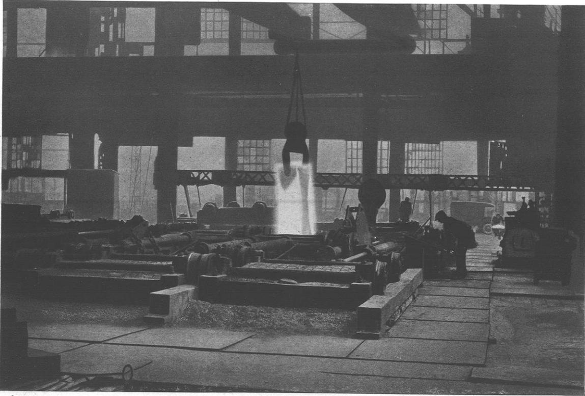
White-hot steel ingot being drawn from the soaking pit. Courtesy of the United States Steel Corporation
