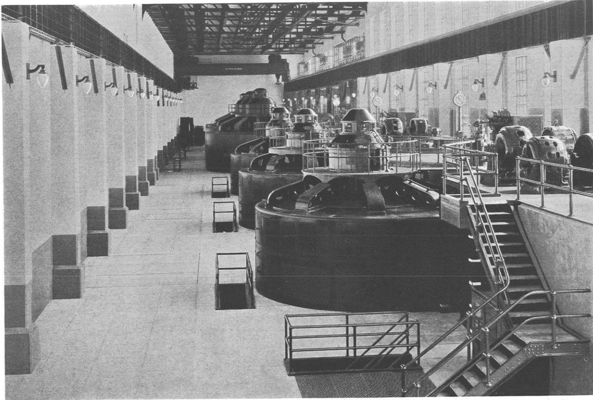
Niagara Falls. Interior of Schoelkopf Station. Three 37,500 h.p. generators in the foreground, three of 70,000 h.p. at the rear. Courtesy of the Niagara Falls Power Company
