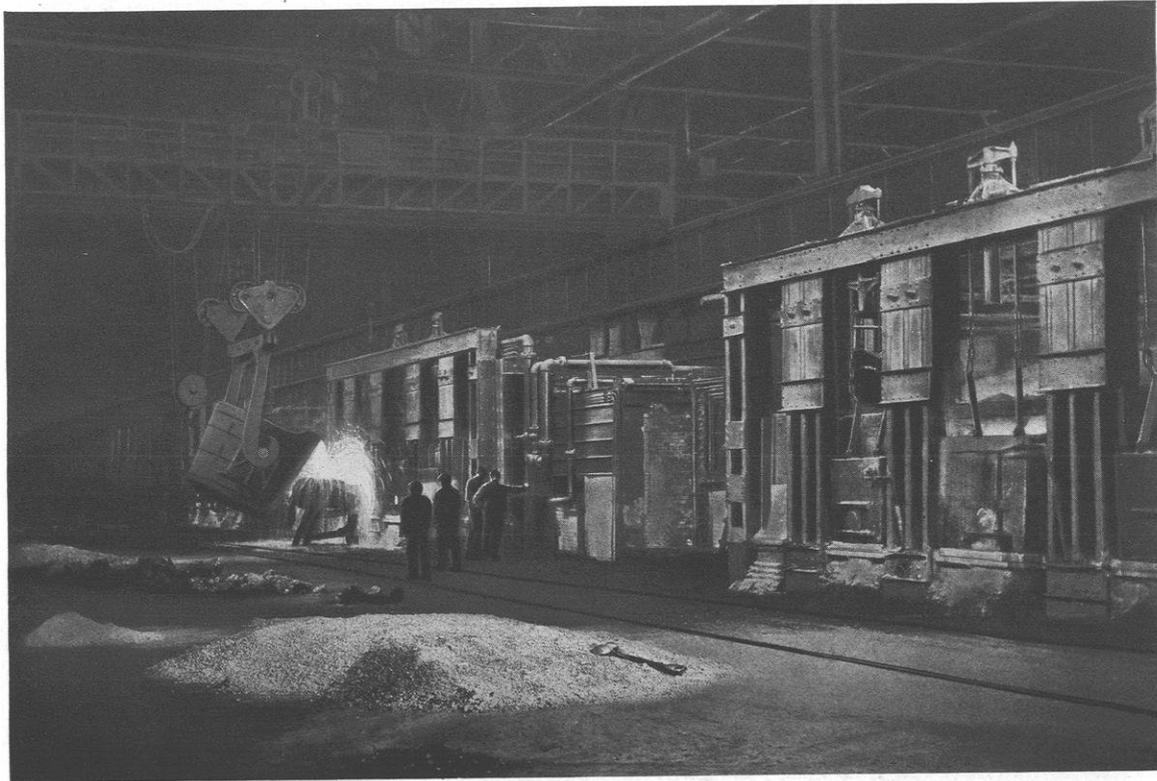
Charging side of an open-hearth furnace steel plant. Courtesy of the United States Steel Corporation
