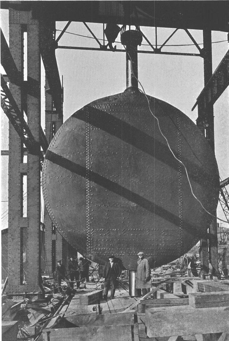
Niagara Falls. Butterfly valve to control water flow. Courtesy of the
