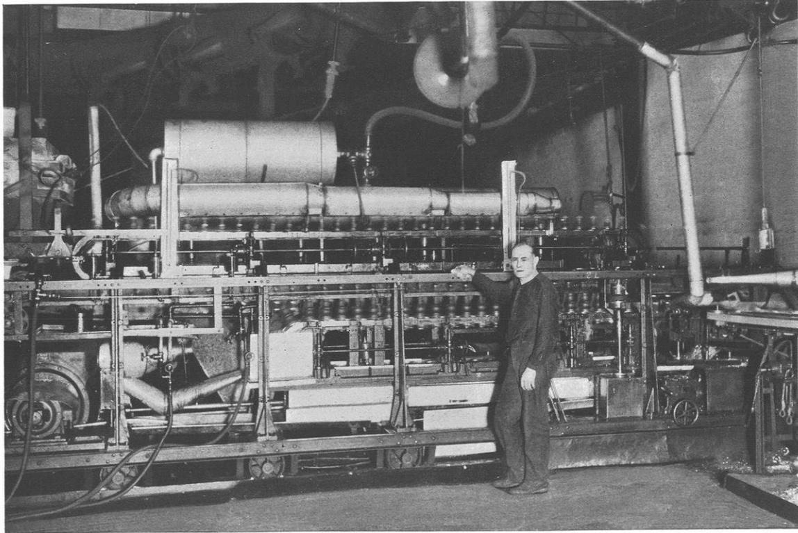
Incandescent light bulb machine. Blows 400,000 bulbs per day. Courtesy of the Corning Glass Works
