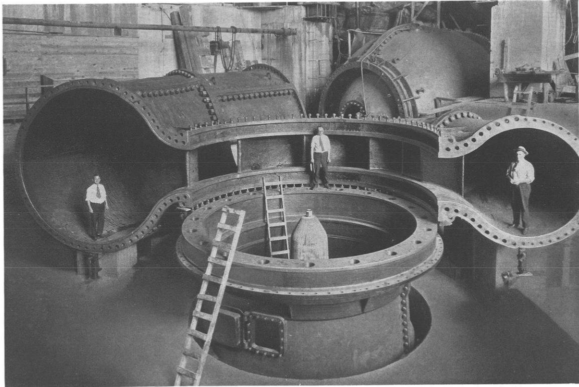
Niagara Falls. Castings being assembled to form wheel casing. Diameter of left-hand opening 15 feet. Whole diameter 47 feet. Penstock shown in the background. Courtesy of the Niagara Falls Power Company
