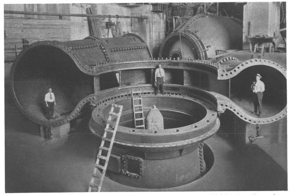
Niagara Falls. Castings being assembled to form wheel casing. Diameter of left-hand opening 15 feet. Whole diameter 47 feet. Penstock shown in the background. Company
