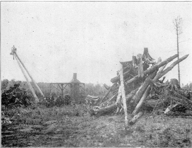
FIG. 2. THE STEAM PULLER WITH ATTACHMENT FOR PILING STUMPS IN HUGE HEAPS.
