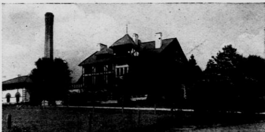
The Dairy Building
