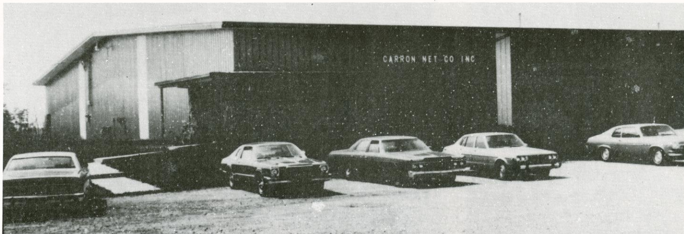
The Carron Net Company built a second plant facility in 1976 and 1977 so large nets could be made indoors. Prior to that, this work was done outdoors and was governed by weather conditions. The large space indoors allowed the company to increase production and provided more room for twisting machinery to manufacture cordage. The plant is located at 2200-27th Street on six acres of land near the West Twin River in Two Rivers. Photo appeared with an article about the company in the Herald-Times-Reporter , July 22, 1979. © Herald Times Reporter, reproduced with permission.
