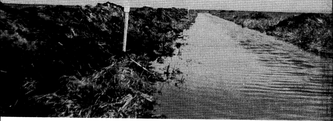
View of portion of ditch following dredging.
