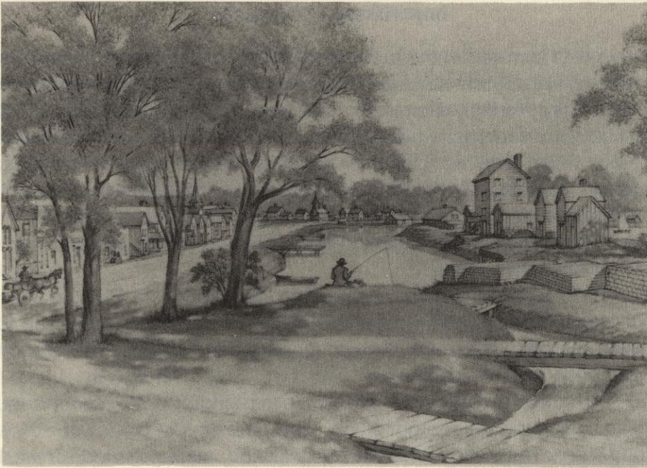
Menasha canal under construction, early 1856.
