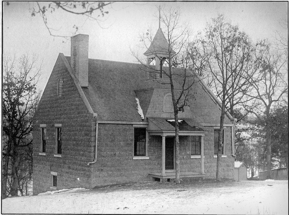
The Malone country school, built in 1905, as it stood before being converted into a private residence.
