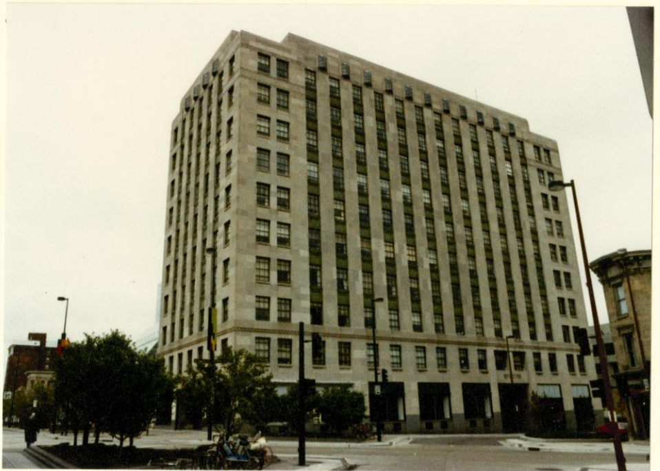
Side facade facing south from E. Main St. Note main entrances to offices on this side.
