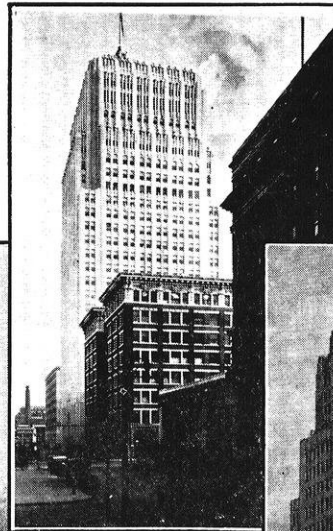
Pacific Telephone & Telegraph Company, San Francisco, Cal. J. R. Miller, T. L. Pflueger & A. A. Cantin, Associate Architects
