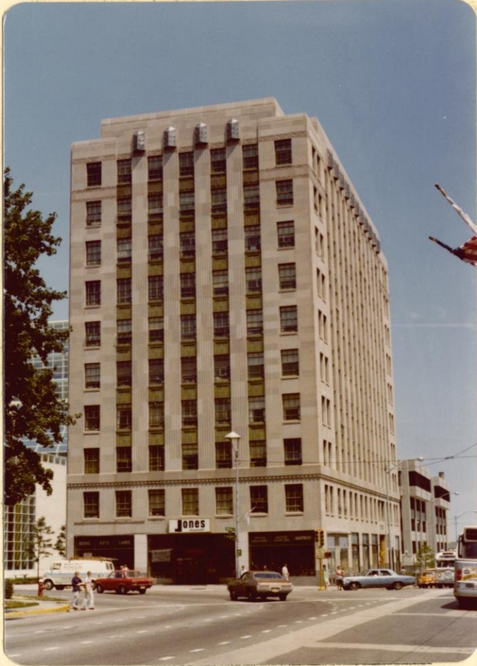
Front facade facing southeast west from Pinckney and E. Main intersection
