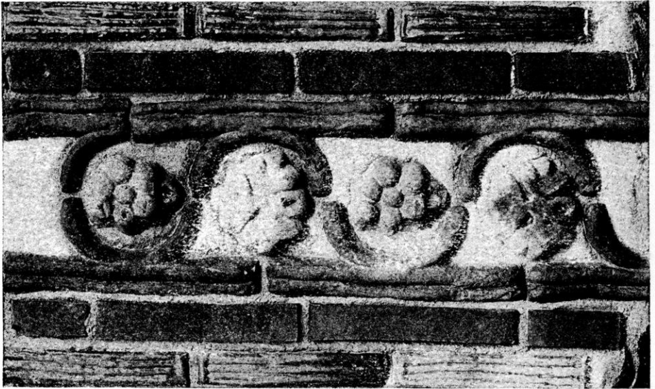
Border of relief tiles set in light cement.
