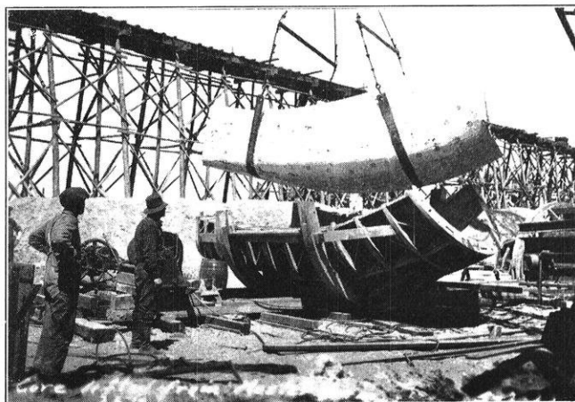
Removing Plaster Cast from Master Pattern
