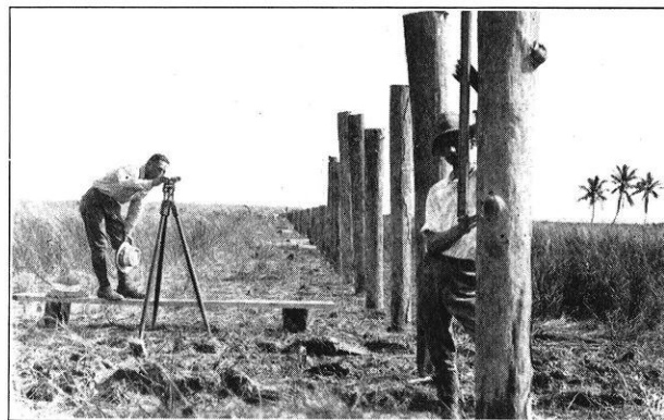
Valuable bay-front property is made by clearing salt water mangrove swamps, and then pumping in sand and rock from the bay bottom. Bulk-heads are constructed on the property lines where necessary.
