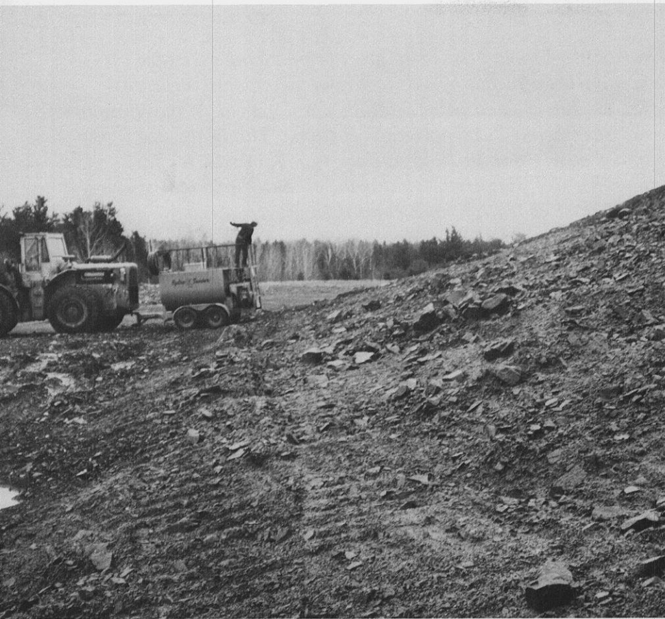
JCIC class 3 ore pile being hydroseeded in May 1981
