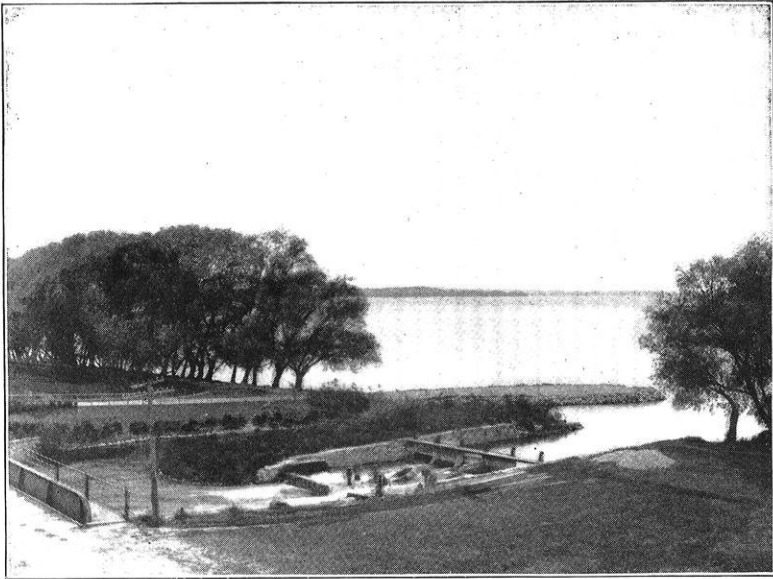
Lock Site Before Improvement.
