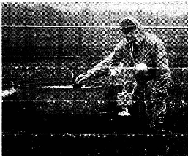
Evaporation pan being monitored by Mr. Hugh Rutherford, the local observer at Vandercook Lake.
