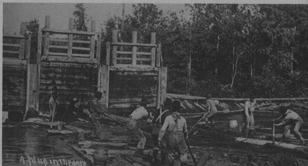
Fig. 3: Close-up of the Dells Dam, Wolf River, built in 1873, 16 feet high and 40 feet long
