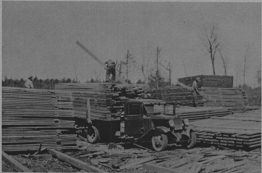
Unloading and stacking lumber.
