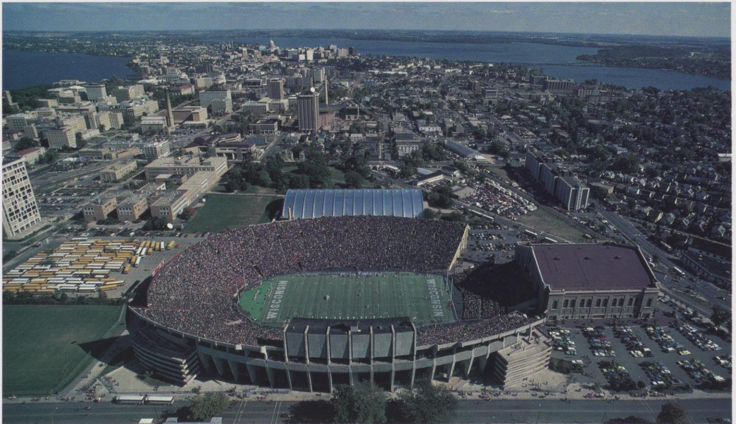
An aerial view of the action—before the construction of the new Dave McClain Indoor Practice Facility.
