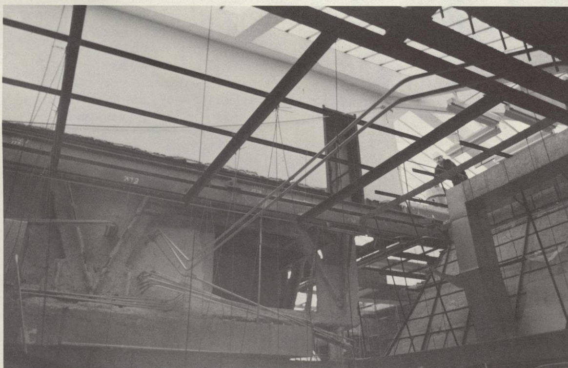
Worker plans procedures to isolate the attic before asbestos-containing fireproof material can be removed.
