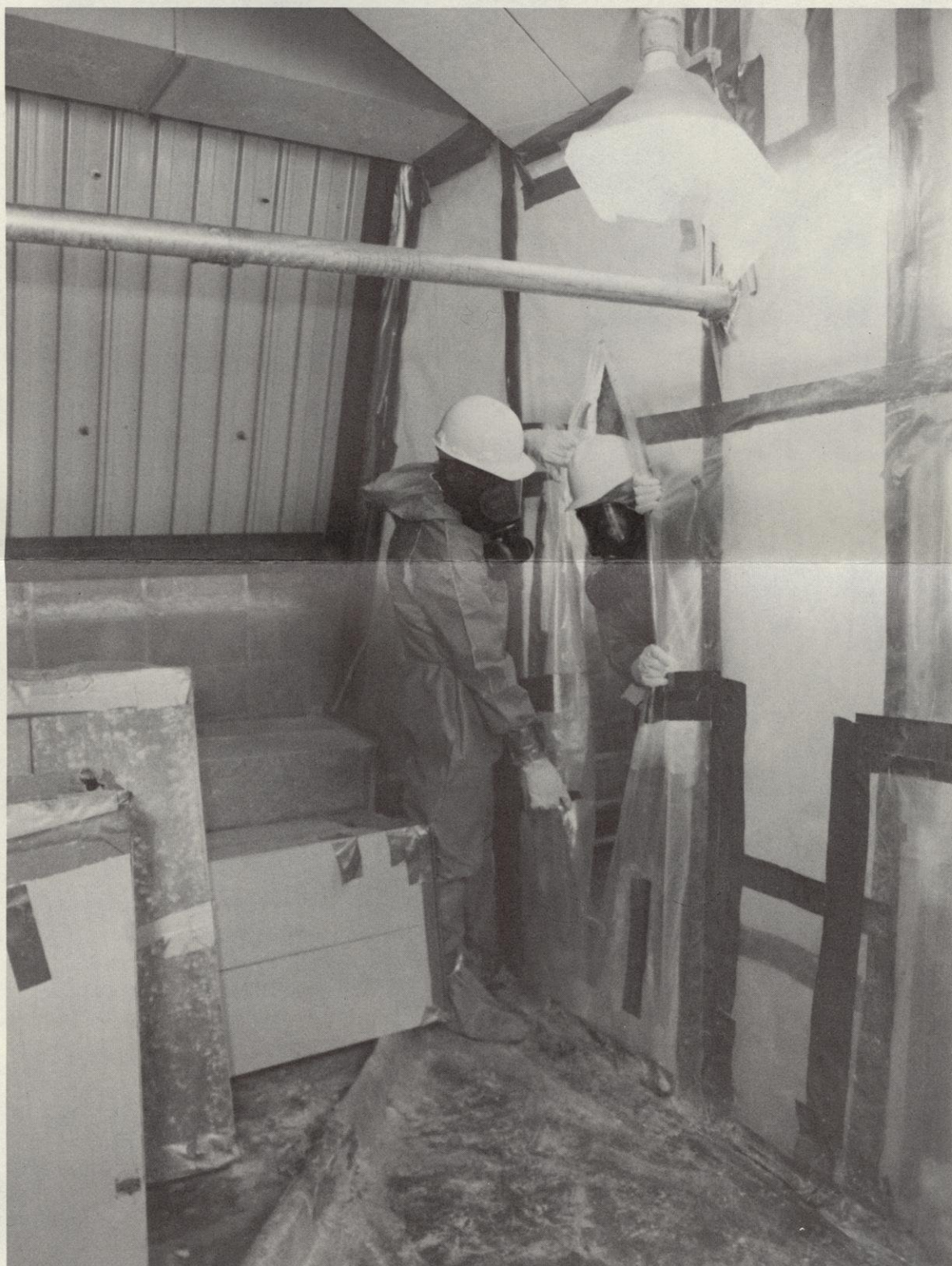
Once the air tests clean, the workers can slice open the critical barrier which isolates the area where the asbestos is being removed.
