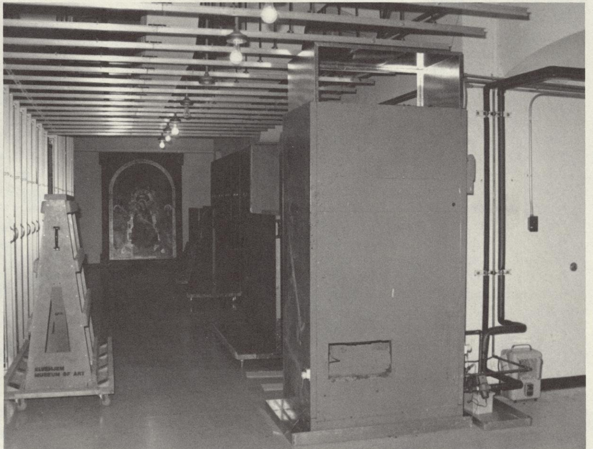
Special heating/cooling units were installed in painting storage.
