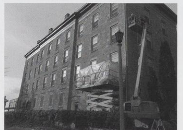
North and South Hall stonework restoration
