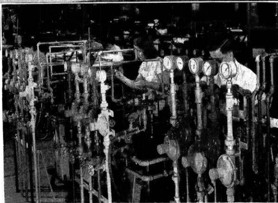
Over 40 miles of pipes deliver 13 needed services to working locations. These are hydrogen, oxygen, nitrogen, city gas, city water, deionized water, soft water (cold, hot, cooling) high pressure air, low pressure air, process steam and condensate return.
