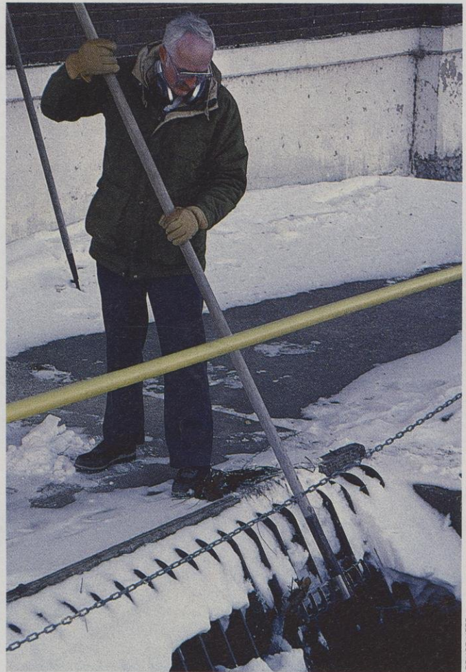
Trash racks in front of a dam act like strainers to keep debris from clogging turbines. Fish can slip through trash racks if the space between the bars is wide enough, but fish and debris may be pinned against the rack by the force of water.
