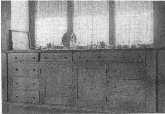
BUILT-IN SIDEBOARD IN THE ROBERTS' DINING ROOM, FILLING THE ALCOVE BENEATH THE WINDOW GROUP.
