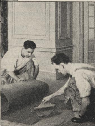
2 Right—One reason why an Armstrong Floor is so warm and comfortable is the warm, heavy layer of builders' deadening felt that is pasted right over the old floor. This felt layer adds quietness, warmth, foot-comfort, and takes up any expansion or contraction of the old wood floor.
