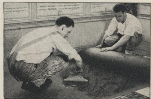
3 Above—Does an Armstrong Floor shrink, expand, buckle? How can it when every square foot is firmly cemented in place? Furthermore, all seams and edges are sealed with water-proof cement—a water-tight, permanent floor.
