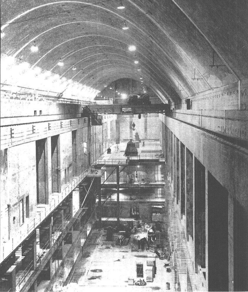
Fig. 3.—275,000 cubic yards of rock were removed from a mountain to make this 700 foot long, 120 foot high powerhouse. Three of eight generators are shown in position.
