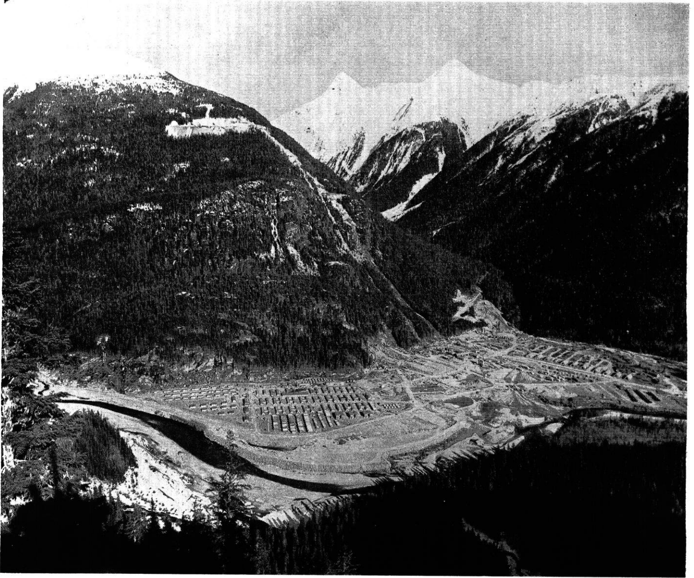
This is the site on the Kemano River (foreground) chosen for the location of the underground powerhouse. It is situated at the level of the construction camp and about 1,500 feet inside the foot of the mountain at the left. The path cleared up the mountain side shows the location of the aerial tramway used to carry men and equipment to the camp 2,600 feet up the mountain. The road beside Horetzky Creek (right background) was built for access to the Horetzky adit, or access tunnel. From this adit, construction was undertaken toward both ends of the ten mile tunnel.
