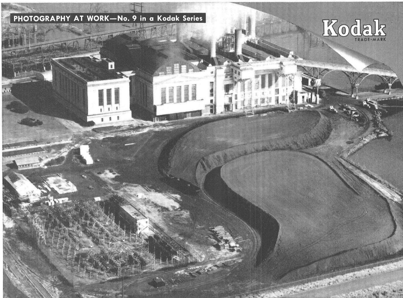
Richmond Station of the Philadelphia Electric Co.
