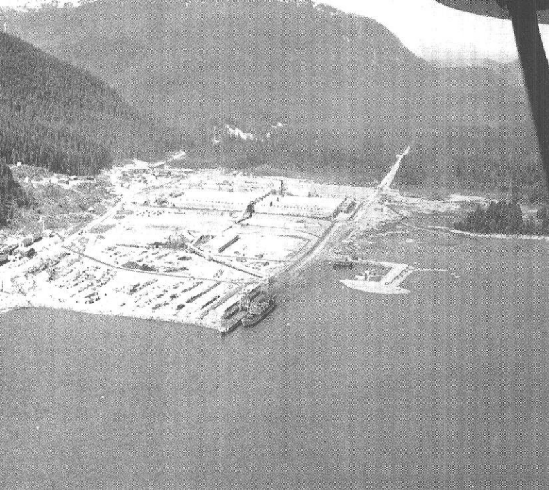
Fig. 5.—At the Kitimat smelter alumina shipped in by boat from Jamaica is refined into pure aluminum. Power used here is generated at the Kemano station 50 miles away.
