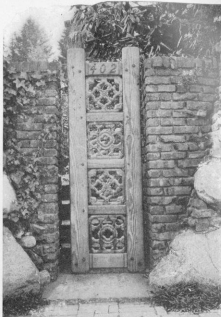
A UNIQUE GATE OF PINE TIMBERS AND COLORED PORCELAIN TILES SET IN A BRICK WALL.
